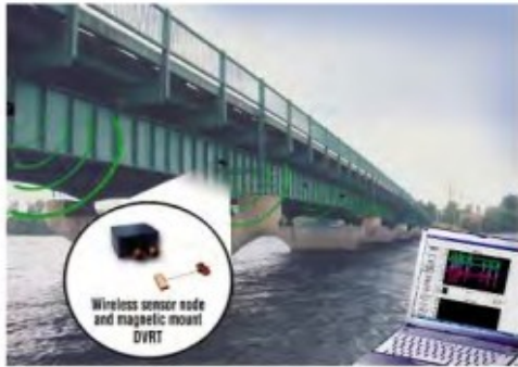
3. Wireless sensors are used to measure long-term stress and strain in civil engineering structures like buildings and bridges. (Courtesy: Microstrain Inc.)
